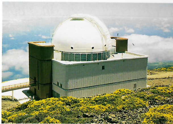
Fig. 2 The observatory building of the Isaac Newton Telescope is protected by a solar screen against direct solar heating. A ventilation system uses the brown painted stairwells to the east and west. White chippings cover the black asphalt around the building, and the yellow flowers indicate the presence of the cordesa bushes which provide a natural solar screen for the rocky terrain. All these factors preserve the natural seeing against convection currents.
