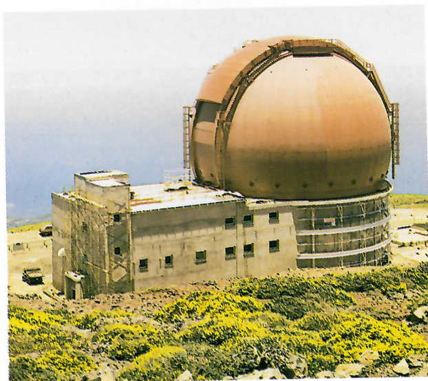
Fig. 2 The Herschel Telescope building nears completion (summer 1985).
