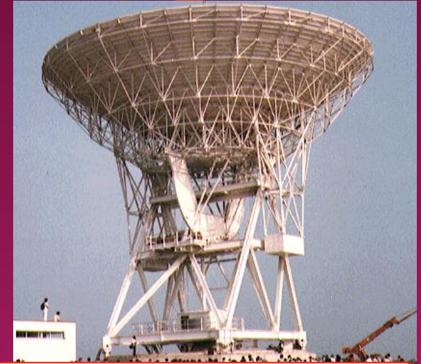
Ground tracking station
