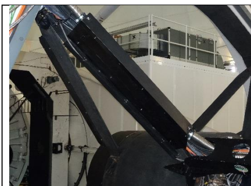
Figure 6 Cable channel on upper left vane
