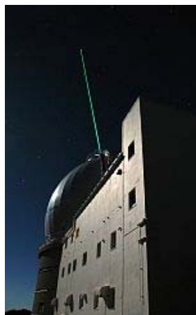
Caption: The GLAS laser beam produces a bright star-like beacon at an elevation of some 15 kilometres above the observatory. This beacon is used to sense the wavefront distortions due to the atmosphere, which are subsequently corrected for with the Adaptive Optics system. Credit: Tibor Agócs.
