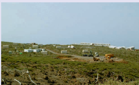
MAGIC foundations close to the former HEGRA site with the Residencia in the background.
