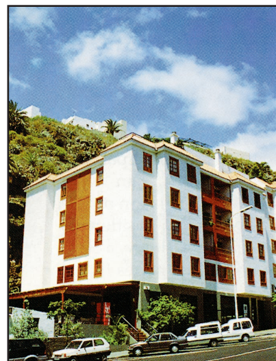
Accommodation in Santa Cruz is usually in spacious flats in apartment blocks such as this one.
