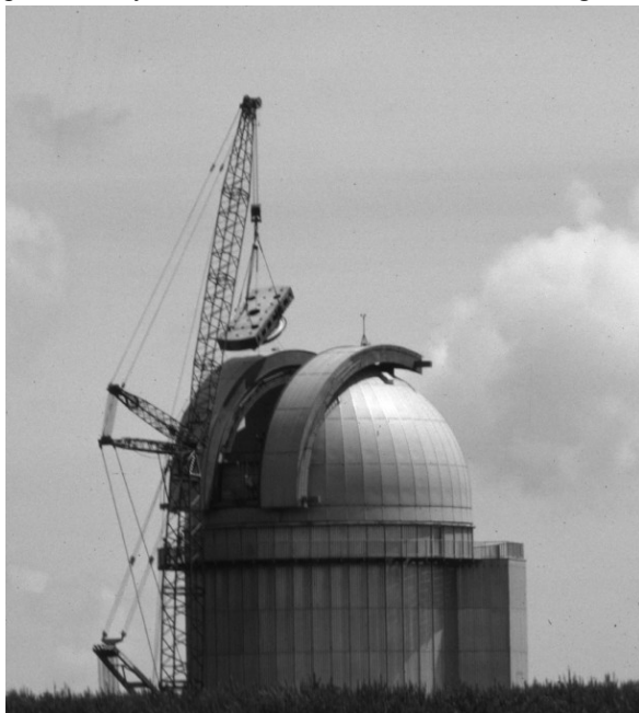
Fig. 2 The INT being dismantled for refurbishment by Grubb Parsons prior to its removal to La Palma.
