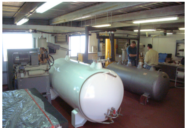
Figure 1. A view of the ING liquid nitrogen plant with the new production unit in the foreground.
