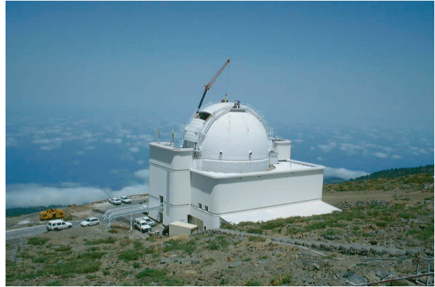
To carry out the work on the INT dome top shutter the largest crane on La Palma was hired to lift the half-tonne units.
