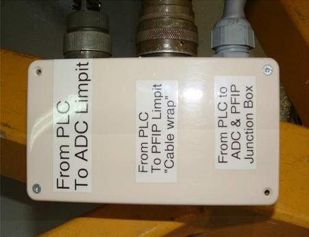
**Figure 2 (PLC connector Plate)**
