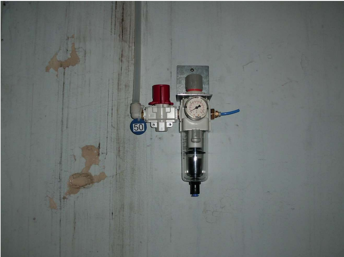
Valve 50 of air supply to the observation floor area of Cassegrain and rolling hose.
