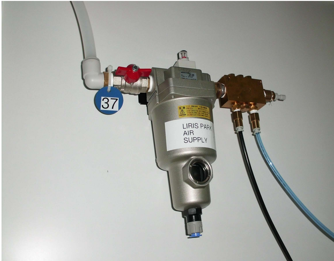
Valve 37 air distributor in the Liris Park room with 1 micron particle filter.
